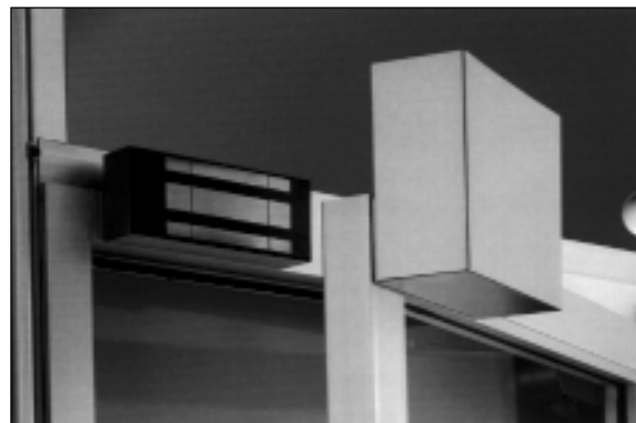
Figure 4-21. Magnetic door lock.
